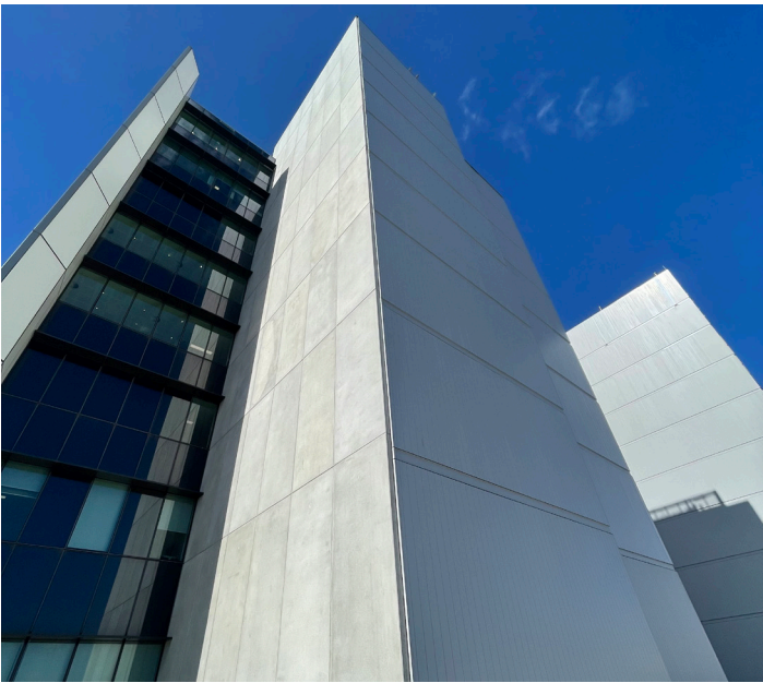
EASTERN EXPRESSED CONCRETE STAIRCORE AND GLAZED STRIP
