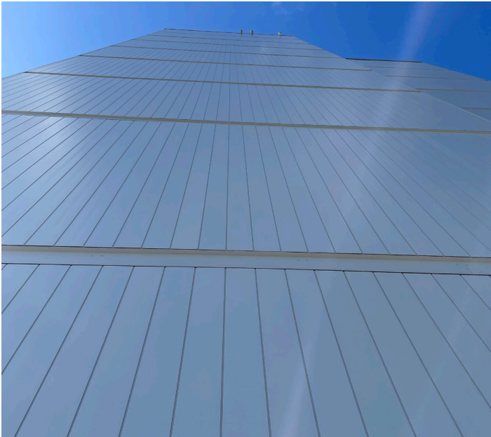
TEMPORARY CLADDING, NORTHERN FACADE
